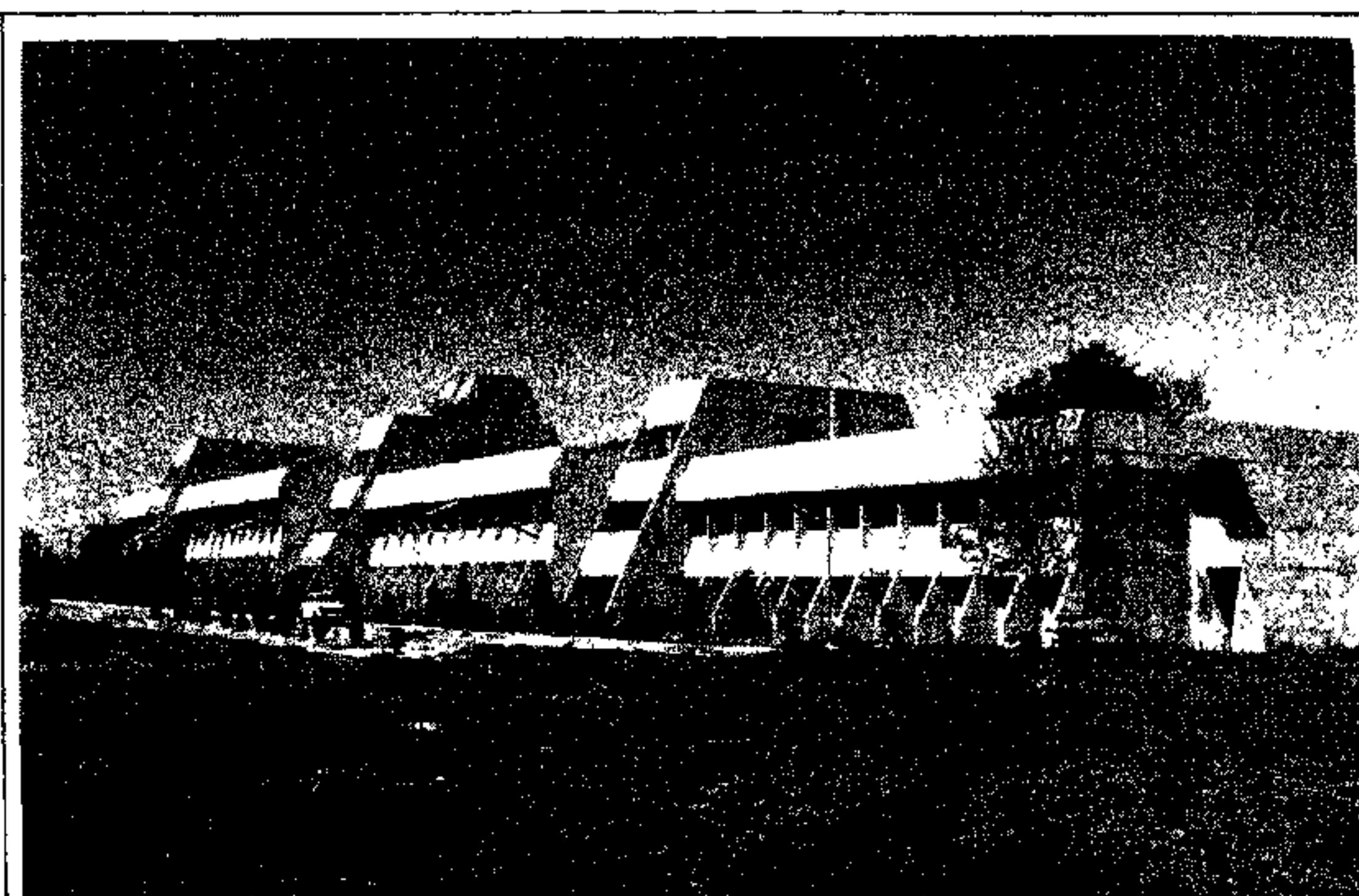
The institute's main building.
