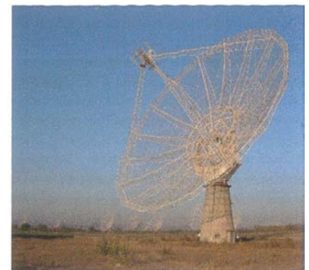
One of the 30 Giant Metrewave Radio Telescope antennas of 45-m diameter: 10 other antennas can be seen in the distance.
