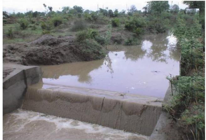
Figure 4. Check dam in the drainage line.
